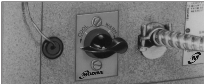
Figure 9.1 - Unit-Mounted Thermostat
