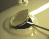
4.4) If an important amount of coating is removed with the cap, repair material can be applied as described further in this document.
