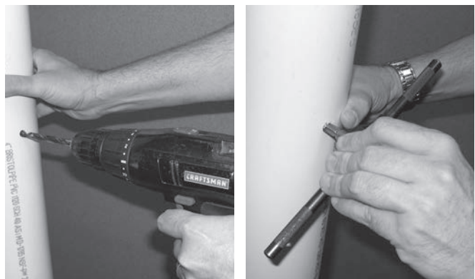
Figure 9.1: Drill and Tap Combustion Test Port
