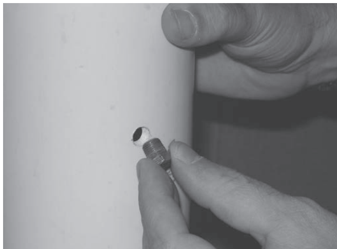
Figure 9.3: Insert Pipe Plug into Test Port
