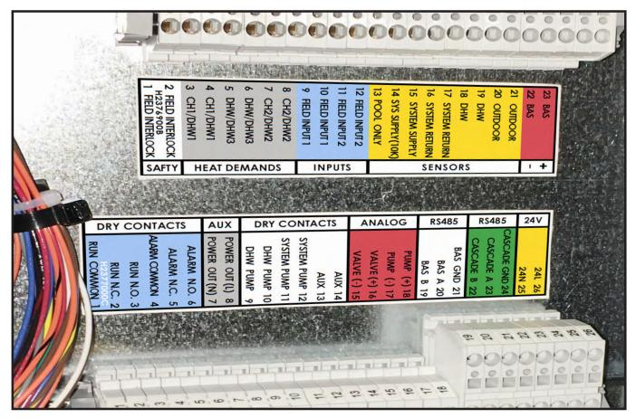
Figure 24. Input and Output Terminal Strips. Low Voltage Connections / Field Wiring
