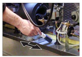
Figure 41. Adjust CO<sub>2</sub> at the air damper
