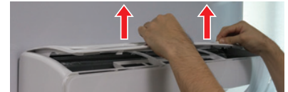
Figure 111: Assembling the Air Filter (Appearances Will Vary Depending on Indoor Unit Model).
