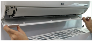
Figure 109: Checking that All Attachment Locations Are Secure (Step 5).
