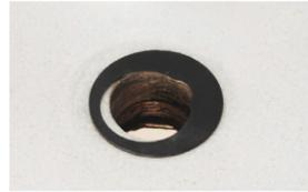
1. Place Counter Gasket over mounting hole to align with profile of dispenser.
