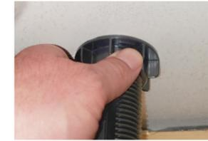
12. Align the Top Assembly above the counter to the desired position and tighten the Mounting Nut against the bottom of counter so the Top Assembly does not easily rotate. Make sure Fiber Optic Cables are not between the underside of the counter and top of Mounting Nut. See Steps 3 and 4.
